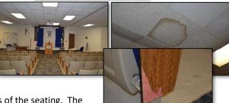
Lecture Hall: The lecture hall has soft tiered seating with carpet tile floor covering at the aisles and the head of the room. There is water damage on some of the ceiling tile that isn't apparent if it is due to an active leak or not.
